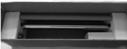
**Step 2:** Ensure the quartz sleeve and UV lamp are thoroughly clean before starting to install. This can be done with alcohol or a mild detergent. Always wear soft non-abrasive gloves to keep any finger marks away from them.
